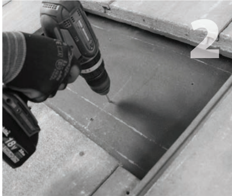
Rest the base plate over center of rafter and mark center of holes. Drill two 7/32" pilot holes and fill with sealant compatible with roofing material.
