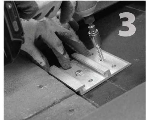
Drive lag screws into rafter through the two holes to a solid, snug fit. DO NOT over tighten lag screws, this may compromise their holding strength.
