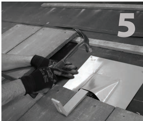
Carefully clean the underlayment, then apply bead of compatible sealant in the shape of an upside down U on the backside of the sub-flashing and install flashing over mount. Fasten sub-flashing to deck with one roofing nail in each top corner. Do not nail bottom corners.
