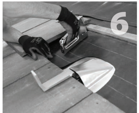
Proceed with weatherproofing using three-course method or lapped paper method.* When using paper method, cut a piece of underlayment 18" wide to slide under the course above and over the sub-flashing. If course above is too high, you must use additional underlayment to ensure proper overlapping.
