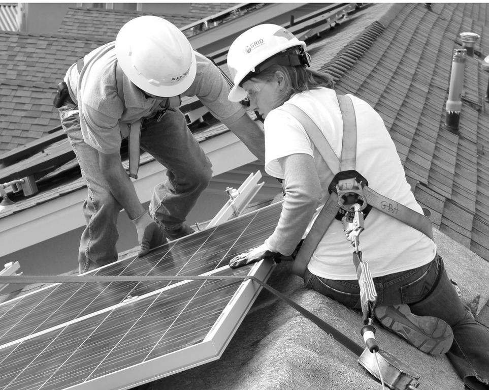
mounted at a fixed angle facing south, west, or east, or mounted on a tracking device that follows the sun, allowing them to capture the most sunlight. Many solar panels combined together to create one system is called a solar array. For large electric utility or industrial applications, hundreds of solar arrays are interconnected to form a large utility-scale PV system.<sup>2</sup>
