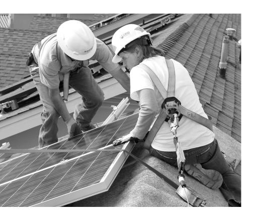
mounted at a fixed angle facing south, west, or east, or mounted on a tracking device that follows the sun, allowing them to capture the most sunlight. Many solar panels combined together to create one system is called a solar array. For large electric utility or industrial applications, hundreds of solar arrays are interconnected to form a large utility-scale PV system. <sup>1</sup>
