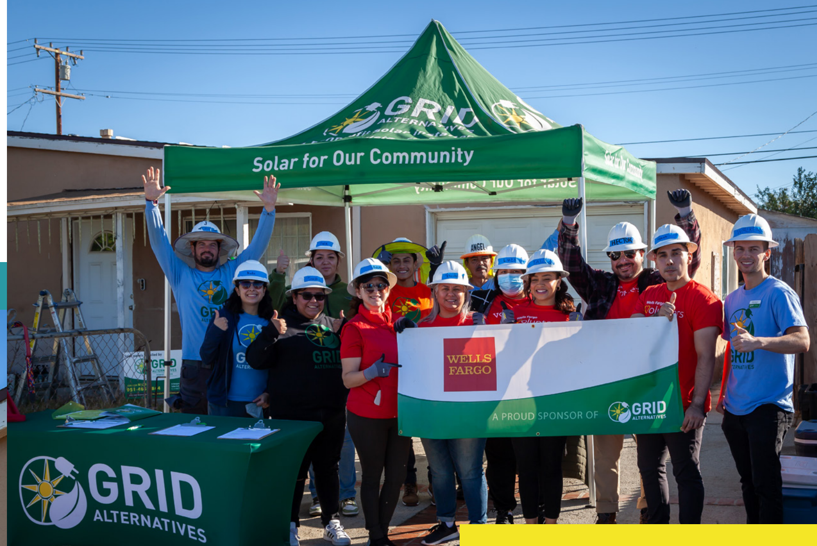
Wells Fargo volunteers installing solar on the Nguyen home in Moreno Valley, California
