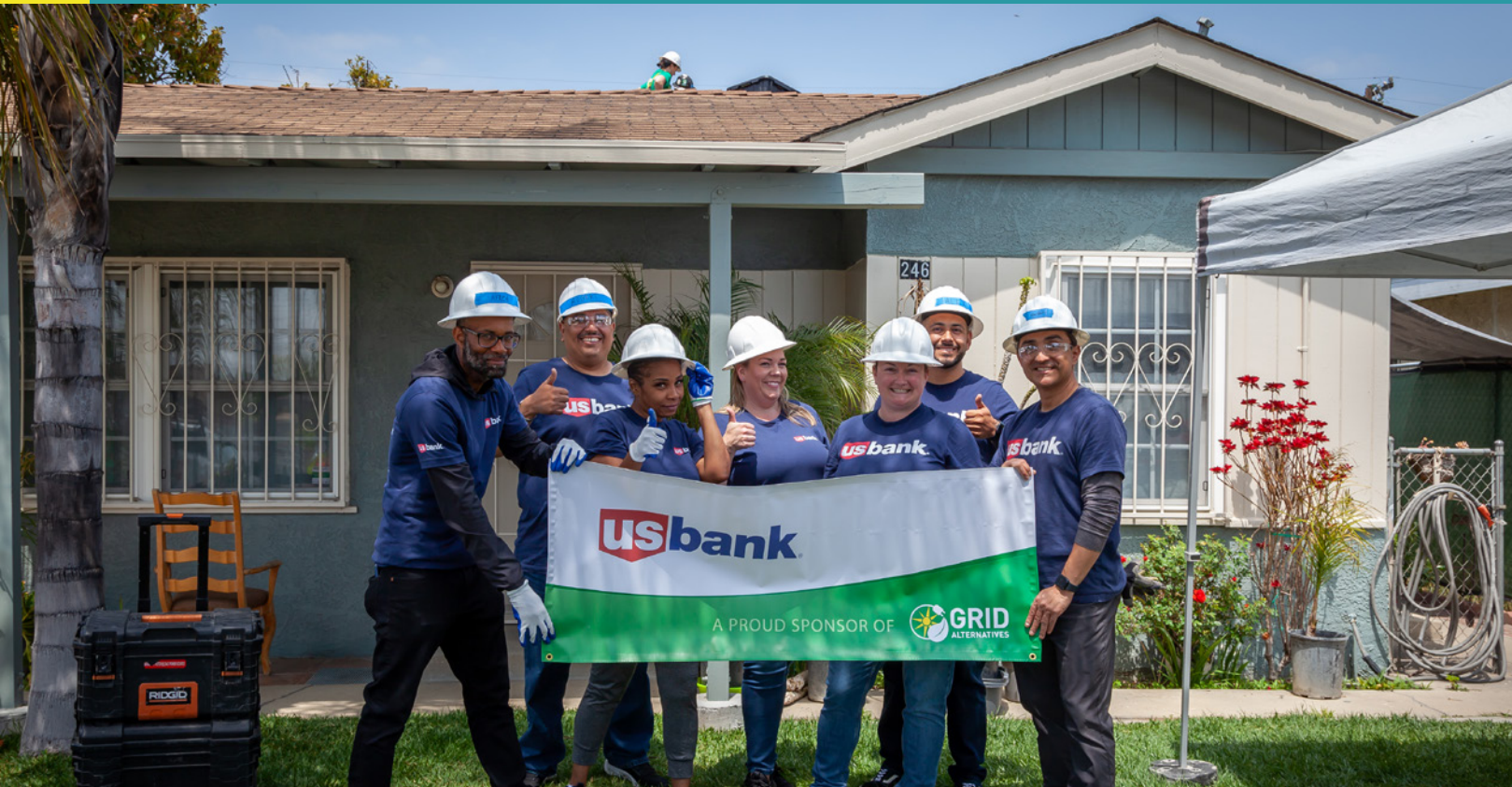
From left to right: U.S. Bank volunteers Alfred, Robert, Lamia, Cassandra, Laurie, Alexander, and Hector, with Katherine up on the roof above
