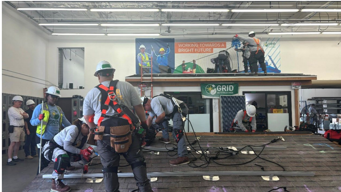
Figure 9. IBT cohort learning PV installation basics (September 2024)
