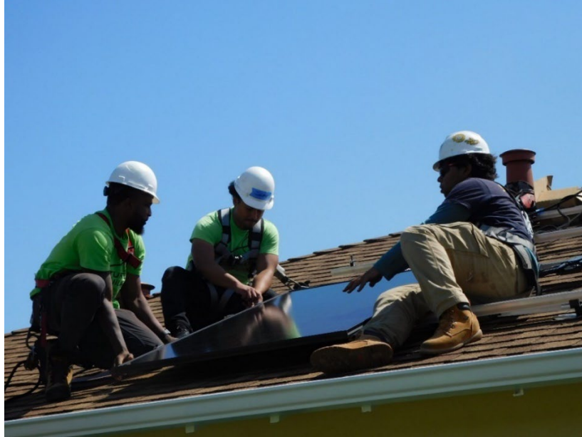
Figure 6. DAC-SASH PV being installed by job trainees in Antioch, CA. (April 2024)
