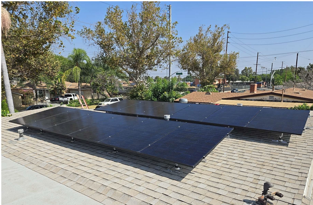
Figure 3. PV array installed by a subcontractor (August 2024)
