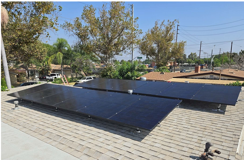
Figure 3. PV array installed by a subcontractor (August 2024)
