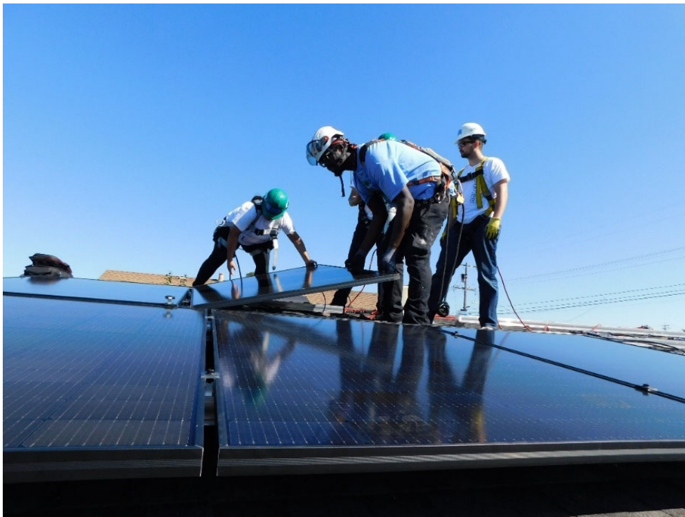
Figure 2. Volunteers installing PV at a DAC-SASH funded installation (October 2024)
