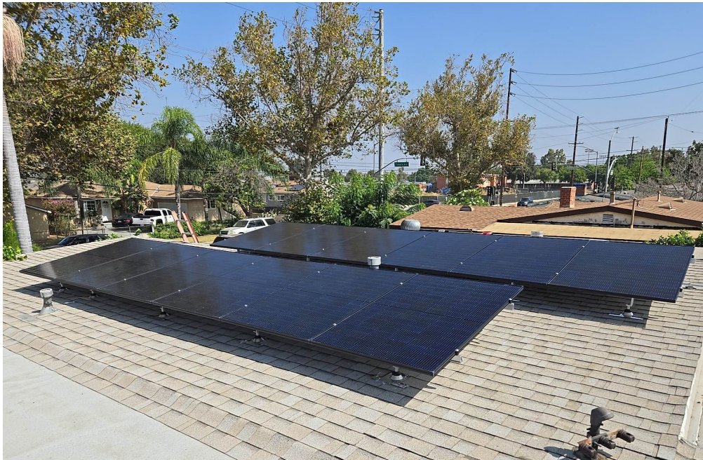
Figure 3. PV array installed by a subcontractor (August 2024)
