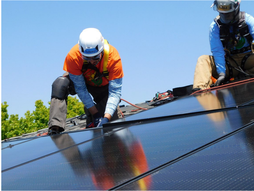
Figure 8. Installation of a PV system (May 2025)
