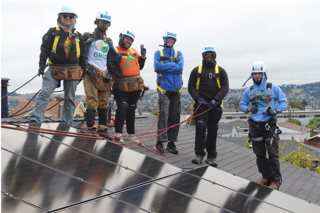
Figure 3. GRID staff installers posing during a PV installation (July 2025)
