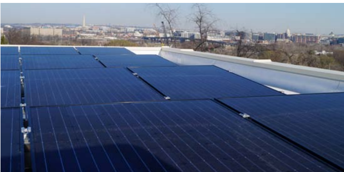
Aigburth Vale is GRID Alternatives Mid-Atlantic's second multi-family project. The first is Parkchester Apartments in Washington, DC.
